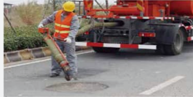
2. Cleaning loose aggregate, dust and water
