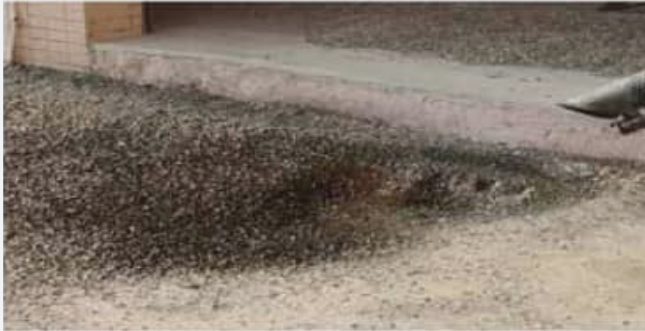
3. Spraying an emulsion layer
