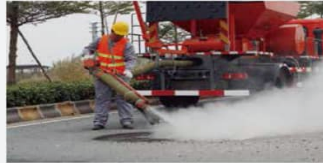
4. Spraying aggregate and emulsion
